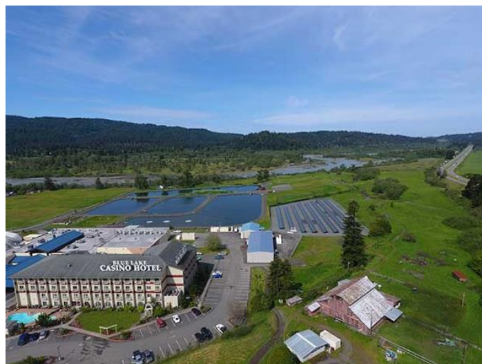
The solar array (right) at Blue Lake Rancheria is part of an innovative microgrid project led by HSU's Schatz Energy Research Center (Photo courtesy of Siemens and Blue Lake Rancheria)
